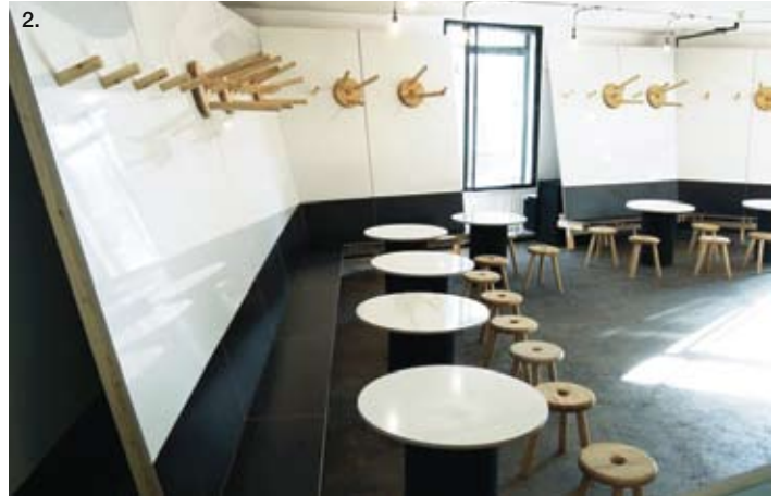
2. Students bar at the Royal College of Art, created from dark brown phenolic film faced birch plywood and white gloss HPL bonded to birch plywood. Courtesy of Markus Bergström.
