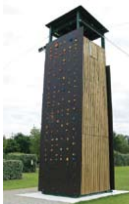
Buffalo® Board used on climbing tower. Photo courtesy of Vid Blakeney.
