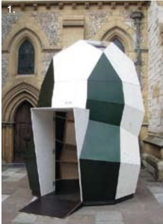
1. Architectural 'POD' installation at Southwark Cathedral London - this was created using a range of ATP plywood, including White Multiwall and dark brown smooth phenolic birch plywood. Created by Tim Greany.
